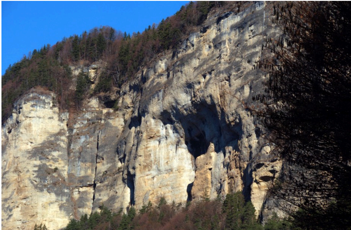
Figure 42: Southern wall of the SC at Kohldorf close to Annabrücke
