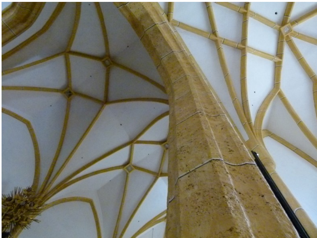
Figure 55: Parish church - ribbed vault, ribs in Nagelfluh — painted.
