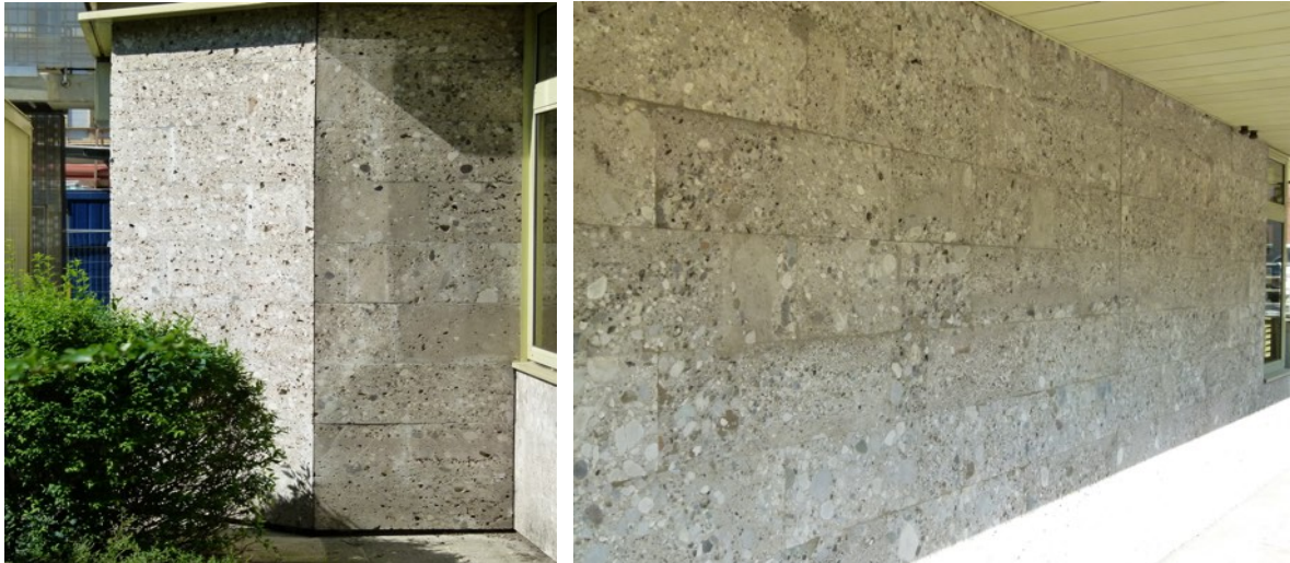
Figure 57: Main Communications Building cladged with SC.
