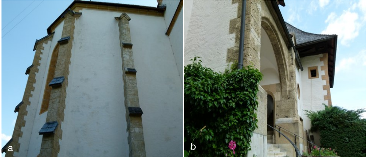
Figure 54: Buttress construction (a) and portal (b), both in Nagelfluh.
